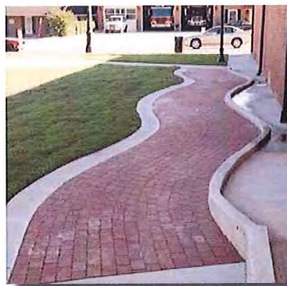
Above: This hexagon paving pattern helps to identify walkways. Below: This sidewalk has a serpentine form to it, carving out space for the adjacent building's stormwater runoff.
