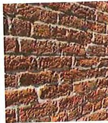
Sandblasted brick surface
