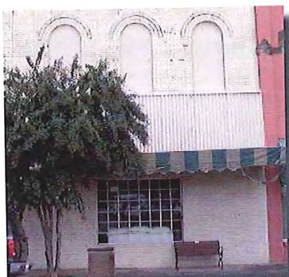
The original arched windows on this building have been bricked in. Re-installing new windows within the original openings is recommended.
