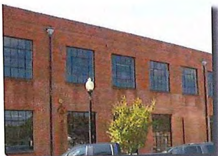
Early industrial buildings often had numerous windows to bring natural light into the interior work space. If any original windows remain, they should be repaired if possible. Replacement units should match the originals.
