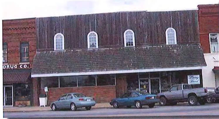
A renovated storefront with inappropriate multi-paned colonial-style windows, wood paneling and shingled awning.
