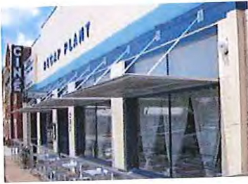
Flat metal canopies are designed to provide cover from sun and rain. Buildings such as the one on the left have brackets which anchor the canopy to the facade. Historic metal canopies should be preserved if possible.
